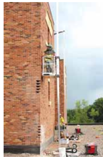
PowerPole PowerTrak drive system uses a 1/2-in. 8-amp drill to lift up to 650 lbs. with a single pole and 1,300 lbs. in a twin pole configuration.
